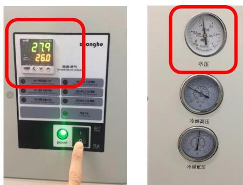
Figure 6-6 T and pressure for water chiller
